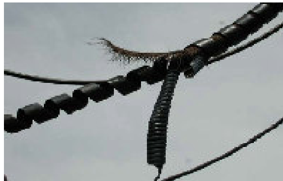
CSB report: ruptured transfer hose
