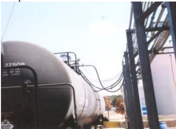
CSB Report: Normal chlorine transfer operations at site showing three 1” diameter transfer hoses
